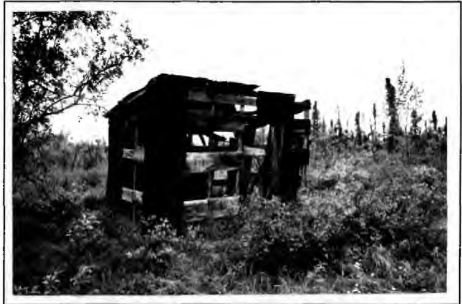
Figure 85. Cap Becker's log and wood frame shed, 1993. The view is looking northeast.
